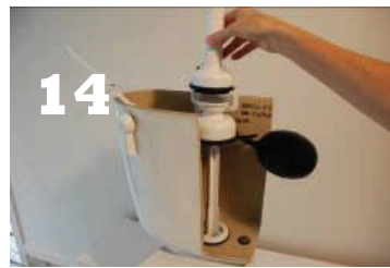
Place entire component over the installed stem.
