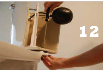
12 Reattach tank to base making sure to push down slightly on tank while tightening bolts for a level snug fit.
