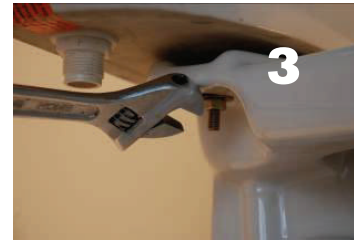
3 Remove just the nuts that connect tank to base Tip: leave bolts in place, it saves a step when reconnecting tank.
