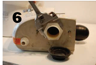
6 Unscrew large nut at base of toilet tank. Remove and discard old valve.
