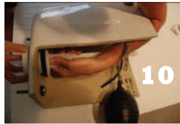
10 Tip10: Push down on valve stem inside tank while reattaching nut. NUT MUST BE VERY TIGHT to ensure a proper seal
