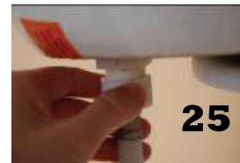
Reattach water supply line and turn on water supply. Check for leaks.
