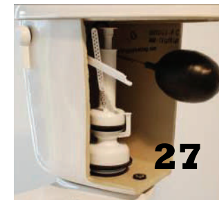
Reattach water supply line and turn on water supply. Check for leaks.
