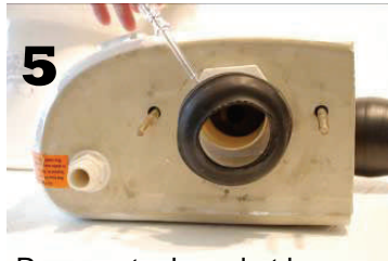
5 Remove tank seal at base (Replace if damaged).
