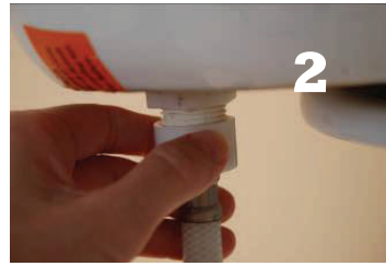
2 Detach water supply line from tank ( Place a towel under the supply line ).
