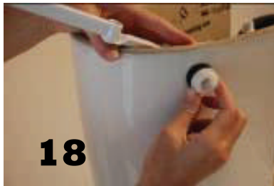
Place lever assembly through tank Re-attach seal and nut. Tighten nut while applying pressure to back plate, this will ensure a tight fit.
